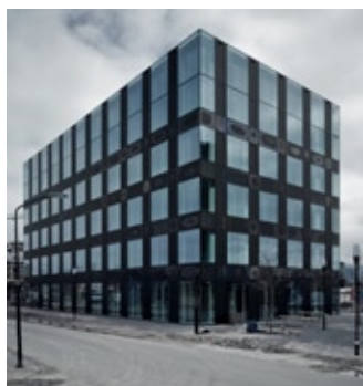
Architecture Dutch Public Prosecution Service ('Openbaar Ministerie'), Lelystad (NL) 2007. Architect: Hootsmans Architectuurbureau
